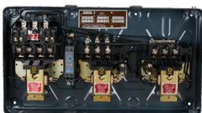
Interior View of MK1 FASD
