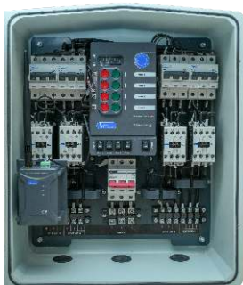
Interior View of xMU-GiA
